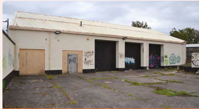
Exterior prior to renovation
