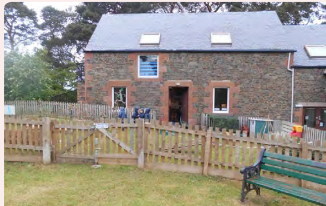
Setting is provided from the community centre which was previously a barn
